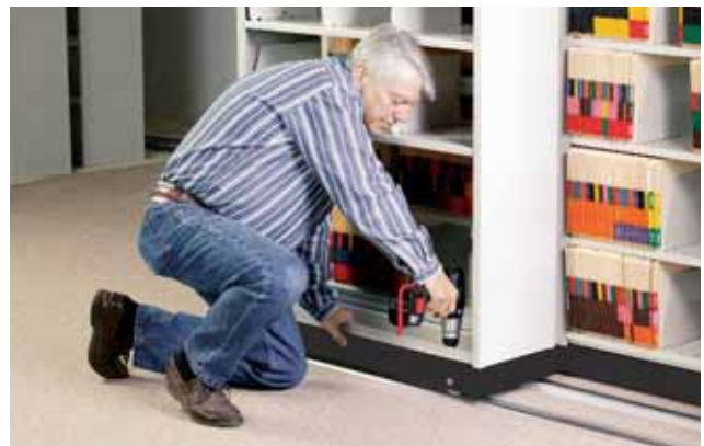
6. Attach shelving to carriage with screws provided.
