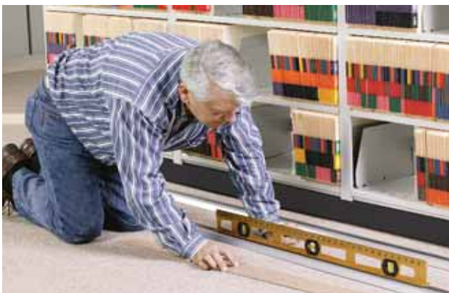
3. Lay down rear track. Check level and shim if necessary.
