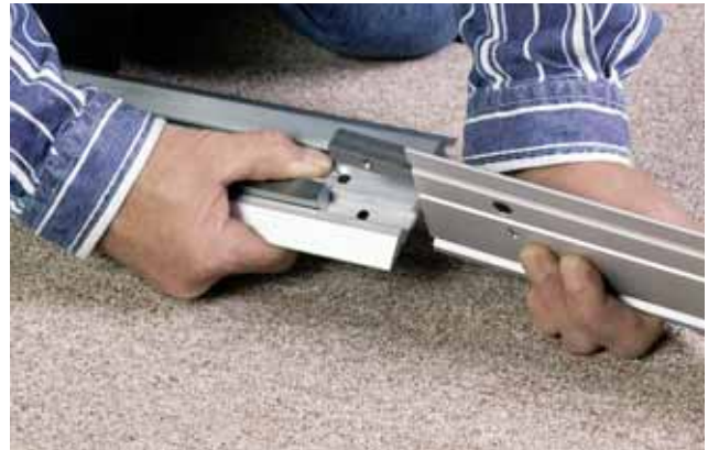
2. Assemble track pieces to system length.
