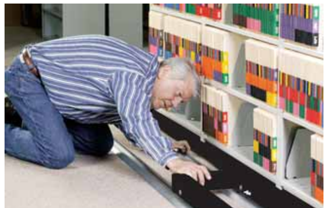
4. Use carriage to set front track. Level, if necessary. Fasten tracks to floor. Attach rear anti-tip brackets to carriages.
